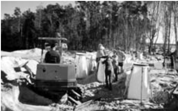
NPWS and volunteers constructed a seawall to protect the Towra Lagoon
