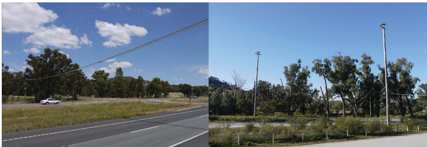
Canopy bridges and glider poles help squirrel gliders cross the Hume Freeway
